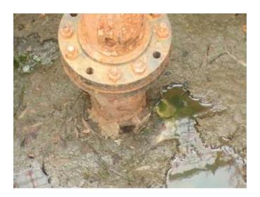
This is clearly a problem. The Companies tell us that once the casing is externally cemented this then prevents Aquifer interchange between one level and another, remove the filling (Cement and or Casing material) and aquifer water will be able to mix between different levels, if this material is eaten away then there is a very great risk of aquifer cross contamination.
