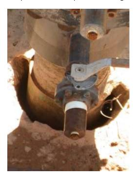
The photograph is of Dewhurst 10 in the PEL238. If the cement is missing at the top where it can be seen, then what is the cementing condition where it cannot be seen? Is the annulus between the inner and outer casings completely filled with cement as the CGS Industry claims?
