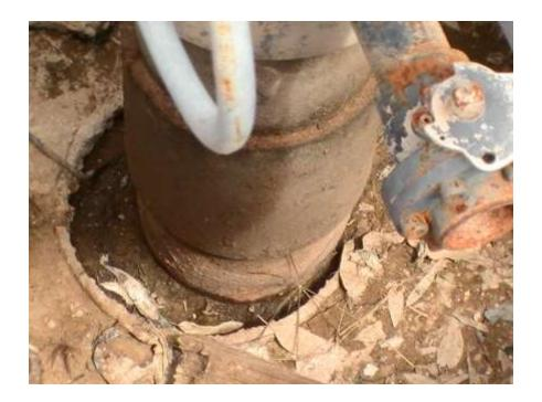
This photo shows Dewhurst 6c clearly off-centre to the outer casing at the very top of the well.
