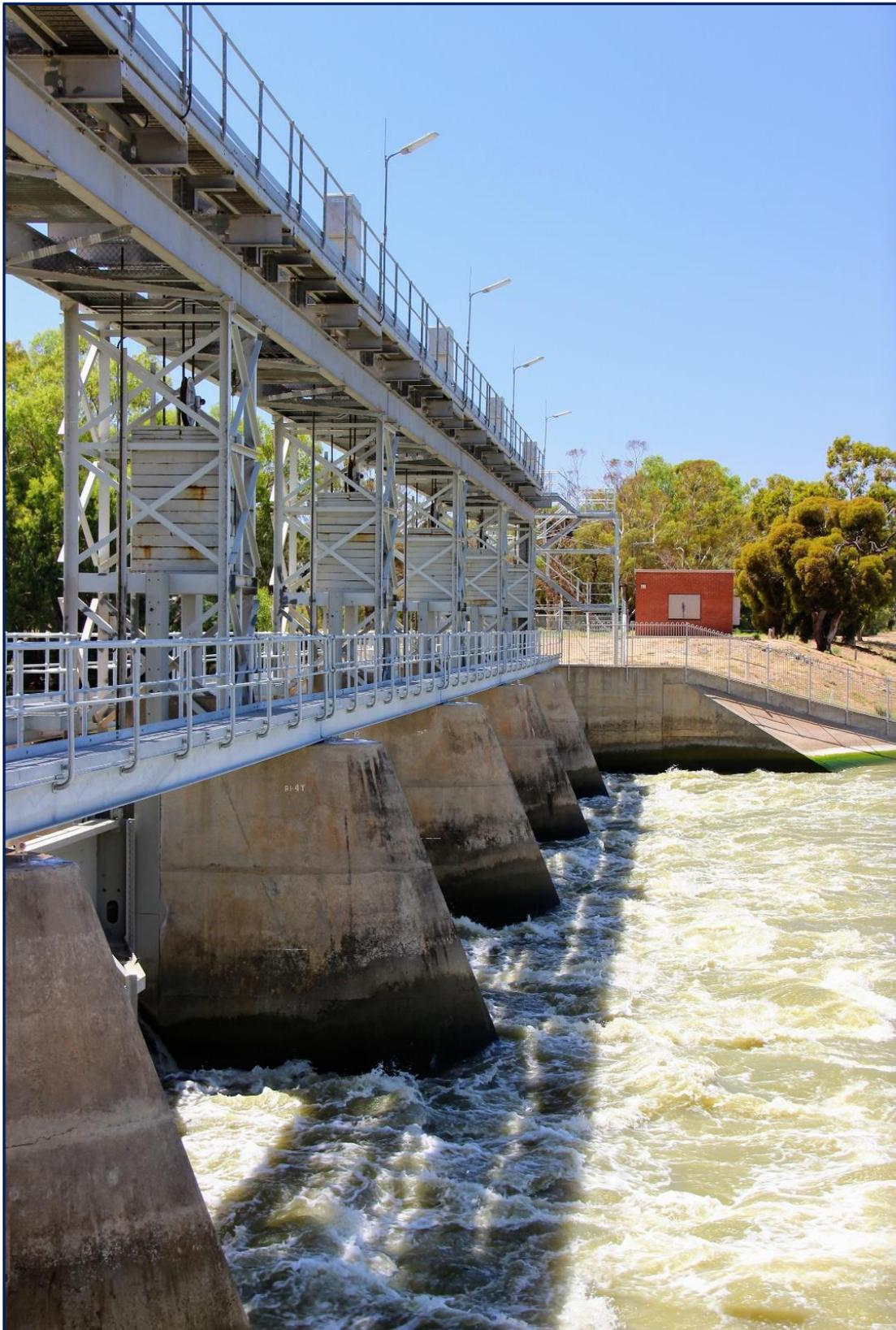
Figure 15-Main Weir, 1 February 2023 releasing ~25,000 ML/d.
